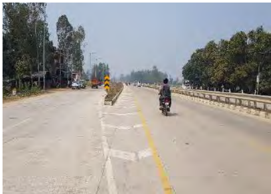
Truck Lay Bye at Km. 37+200
