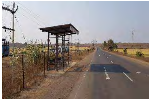
Km. 18+500 – Bus Bay
