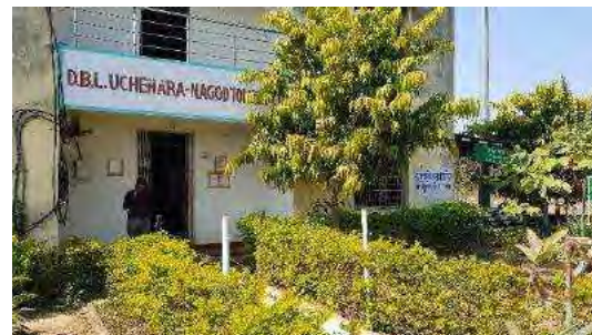
Toll Building at 47+950
