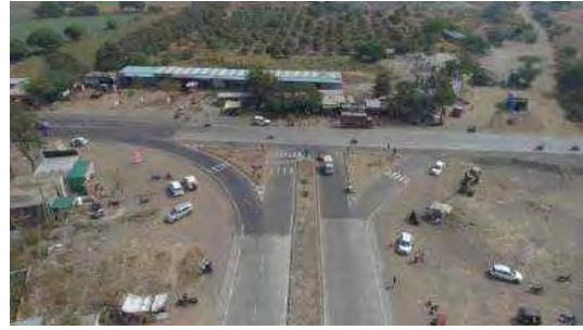
Project End: Km. 55+625
