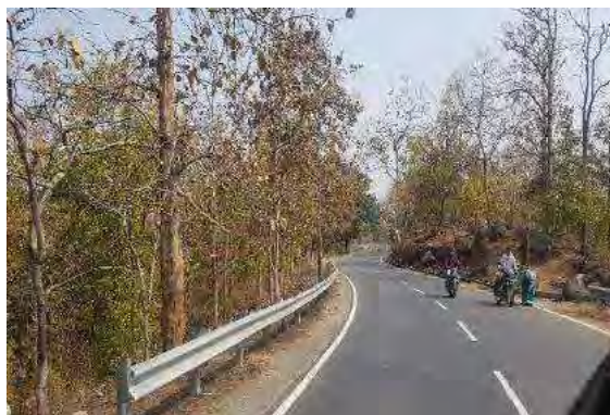
W Beam at approaches at Km.13+300
