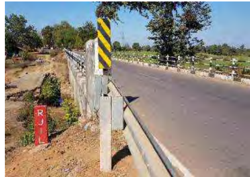
Safety before the Head wall of Box Culvert at 54+610
