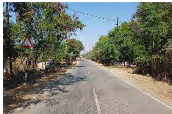
Pedestrian Crossing board at Km. 15+540
