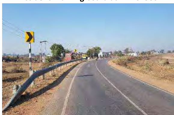
W Beam MCB at approaches at Km. 4+000
