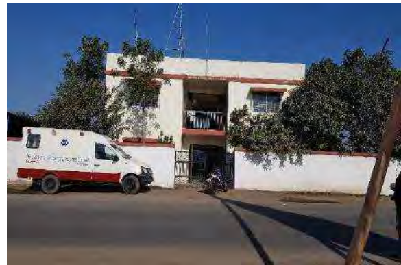
Toll Building At Km.70+000
