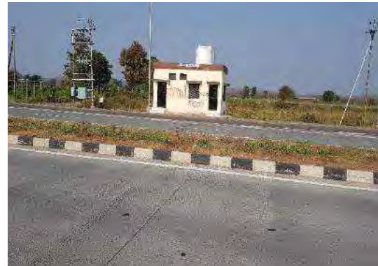
Truck Lay bye at Km.384+300
