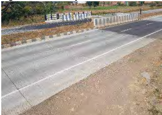
OH marker board before the Head wall at 45+100.
