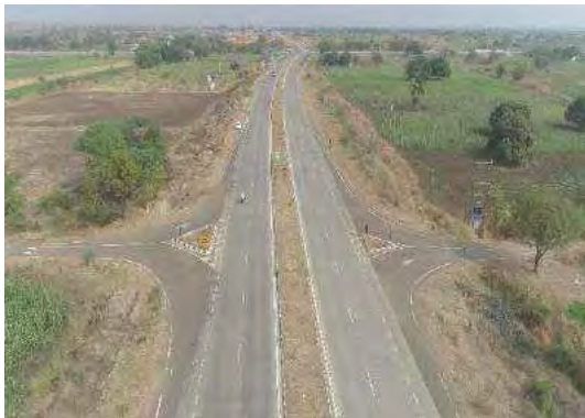
Marking & OH marker at junction islands at Km.2+500
