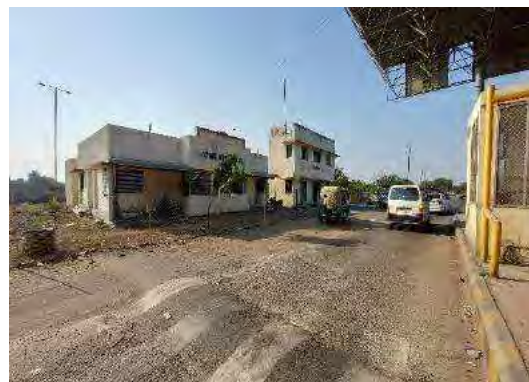
Km. 80+680 at Toll Plaza Figure 7.1 Representative photos of Toll Plaza
