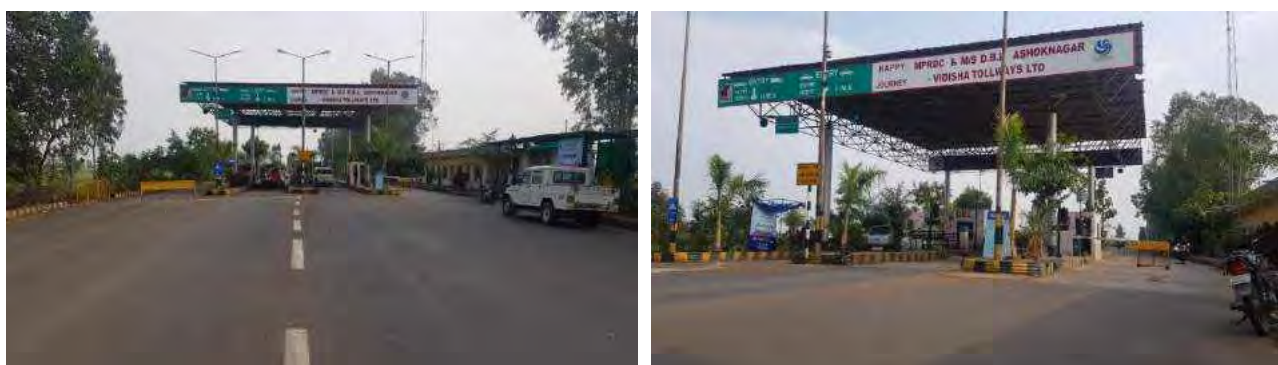
Figure 7.1: Representative photos of Toll Plaza at Km. 7+300
