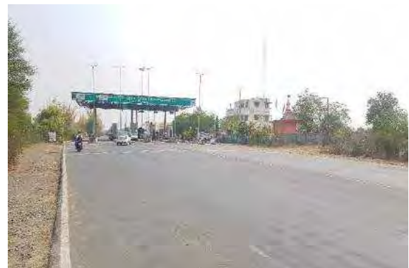
Toll Building at 31+000
