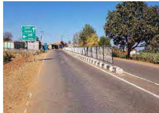
Railing at Builtup sections at Km 55+400
