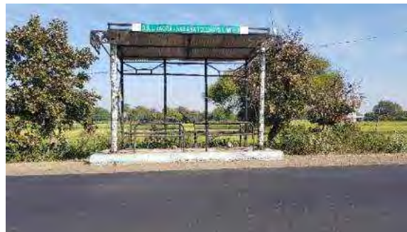
Figure 2.5: Representative Bus shelter at Km. 2+750 of Jaora-Piplodha-Jalandharkheda
