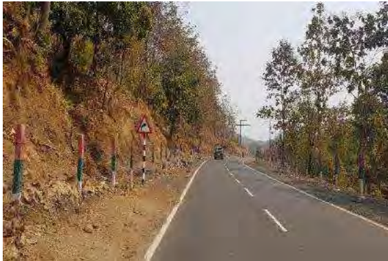
Right Turn board at Km. 76+000
