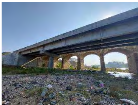
Figure 5.1 Overall view of the Major Bridge at Km 23+611
