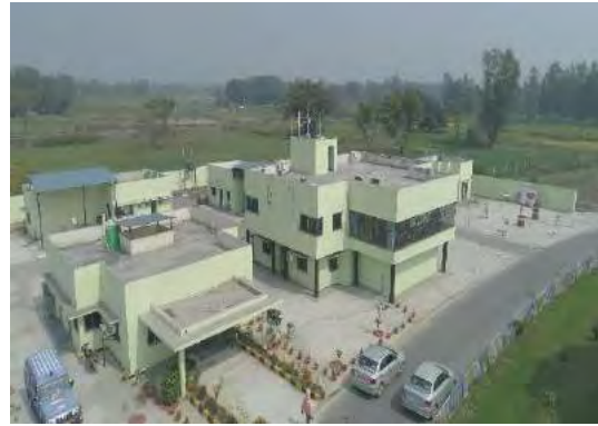
Toll Building Km. 123+490
