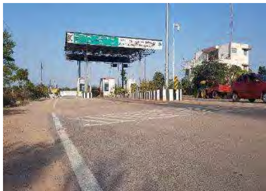
Toll Plaza and Building at Km. 12+000
