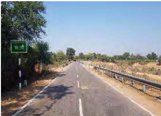
W Beam MCB at approaches of MJB at Km. 28+200
