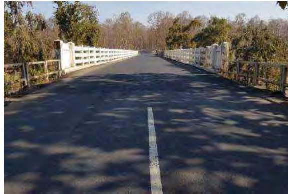
Figure 4.1 : Overall view of the major bridge at Km. 6+841
