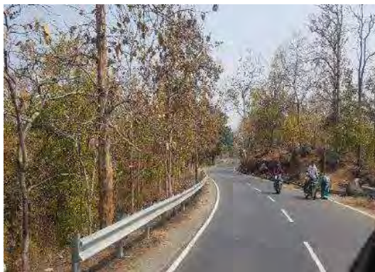
W Beam MCB at approaches at Km.13+500
