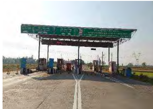
Toll Building at Km. 8+150
