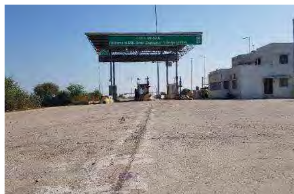
Toll Building at Km. 6+100
