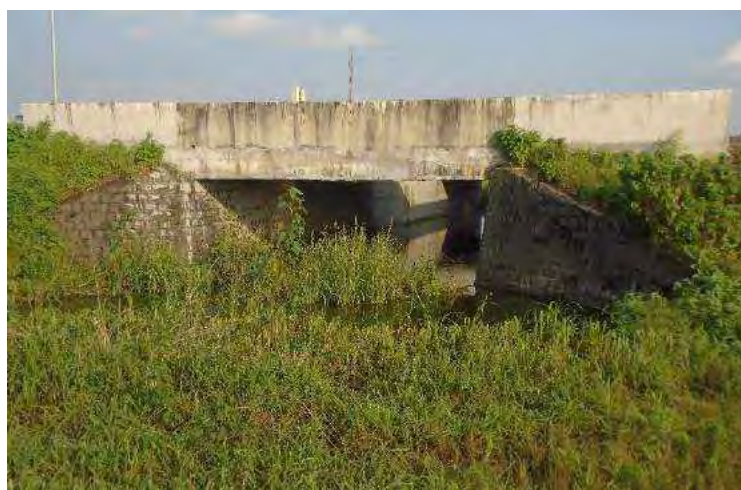
Figure 4.2: Representative photos of Minor Bridges (Km. 289+963).
