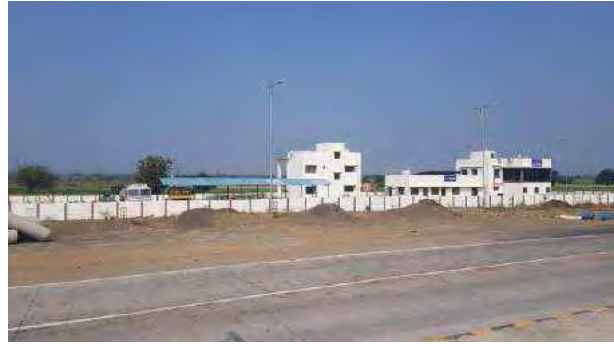
Toll Plaza Administrative Building
