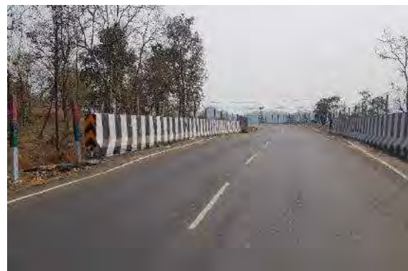
Road safety at the Head wall of Structure at 74+850
