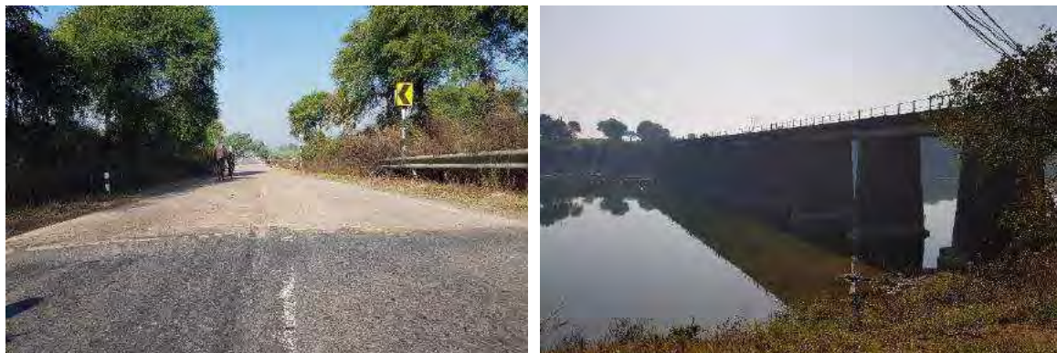
Figure 4.1: Overall view of the major bridge at Km. 4+480
