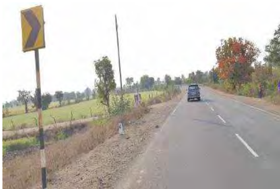
Km. 30+100 – Road Marking
