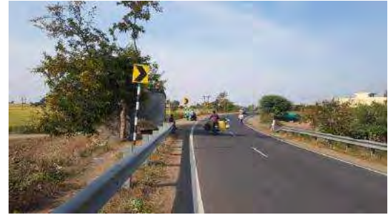
Km. 29+900 Crash barrier at bridge section
