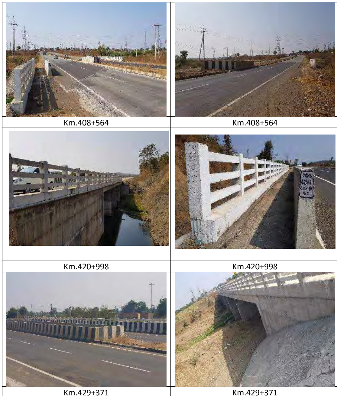
Figure 4-2: Representative photos of Minor Bridges.
