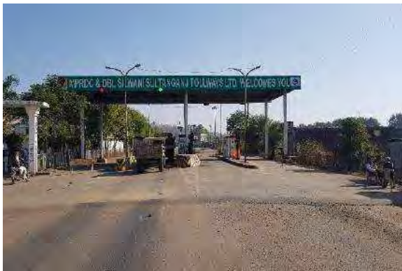
Toll Plaza at Km.70+000
