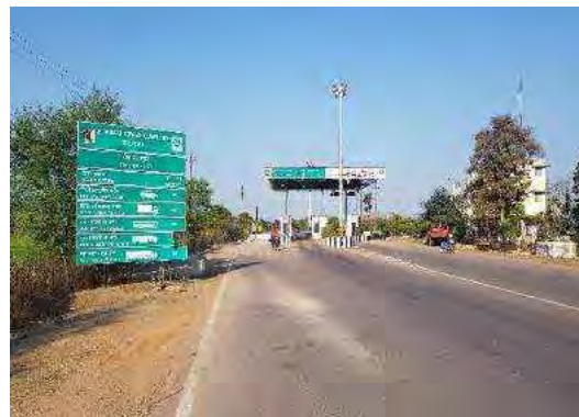
Toll Plaza at Km. 75+900
