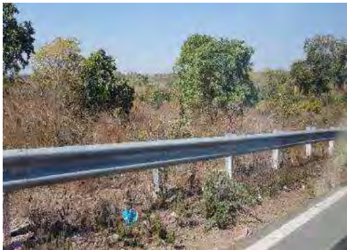
W Beam at approaches of MNB at Km 51+070
