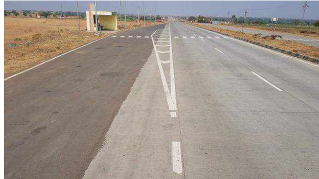
Km. 38+470 Bus bay
