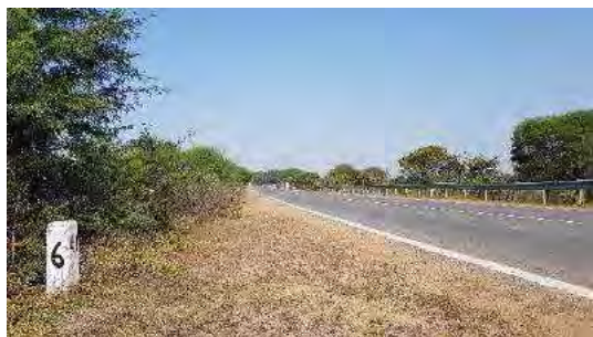
W Beam MCB at approaches of MJB at Km.41+600
