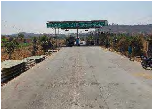
Toll Plaza at Km. 23+800
