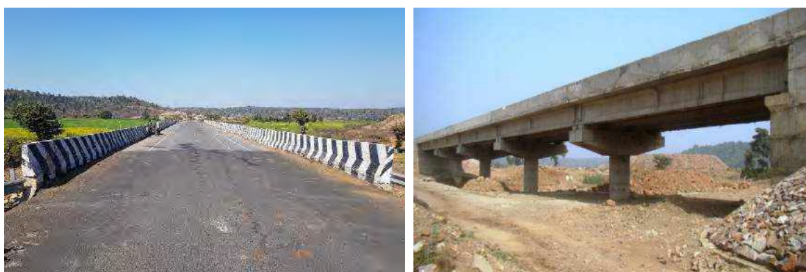
Figure 4.2: Overall view of the major bridge at Km. 40+900
