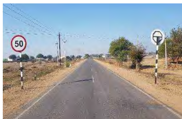
Speed Limit board at Km. 4+000
