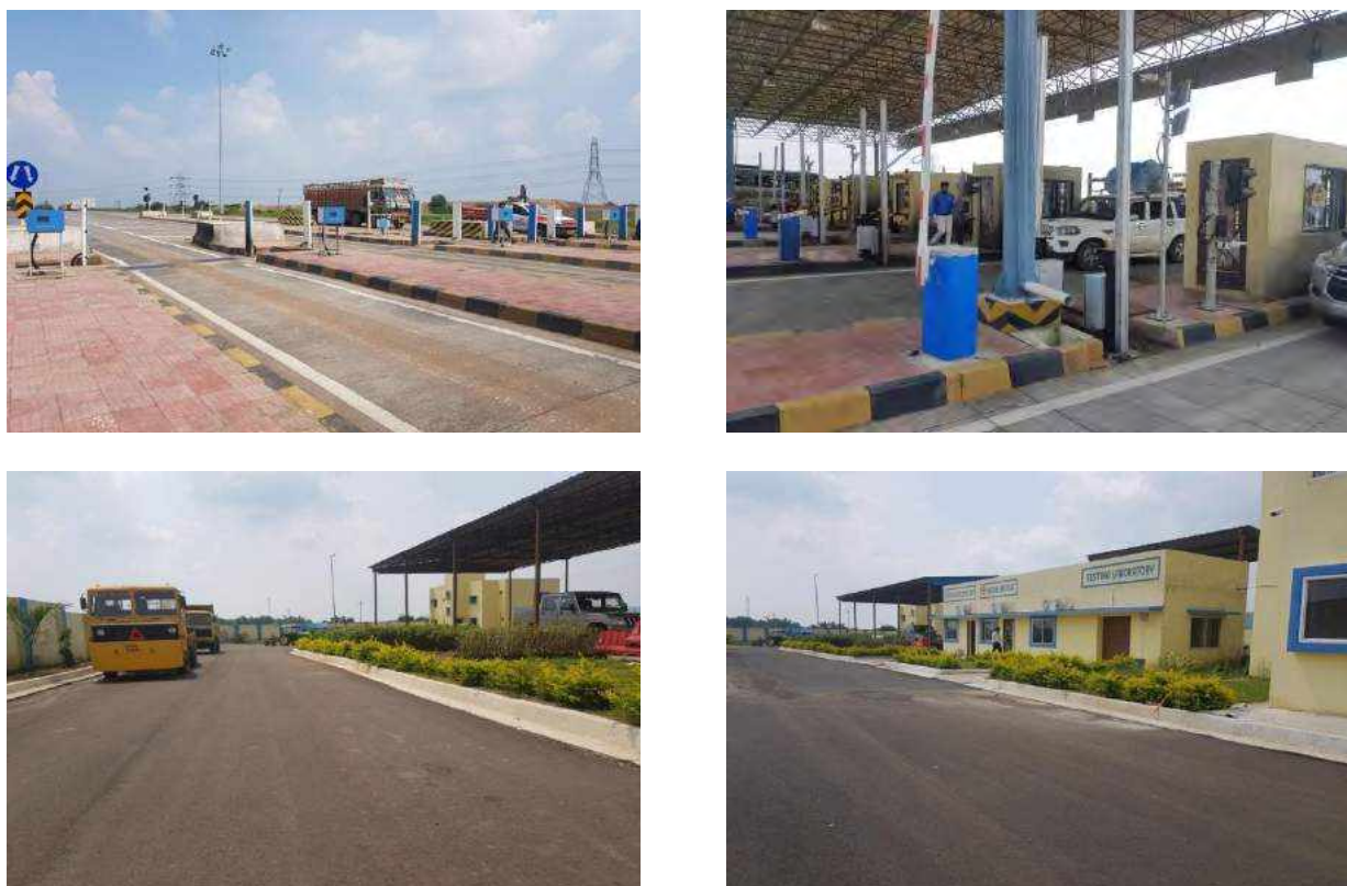
Figure 7.1: Photographs of Toll Plaza at Km. 511+000
