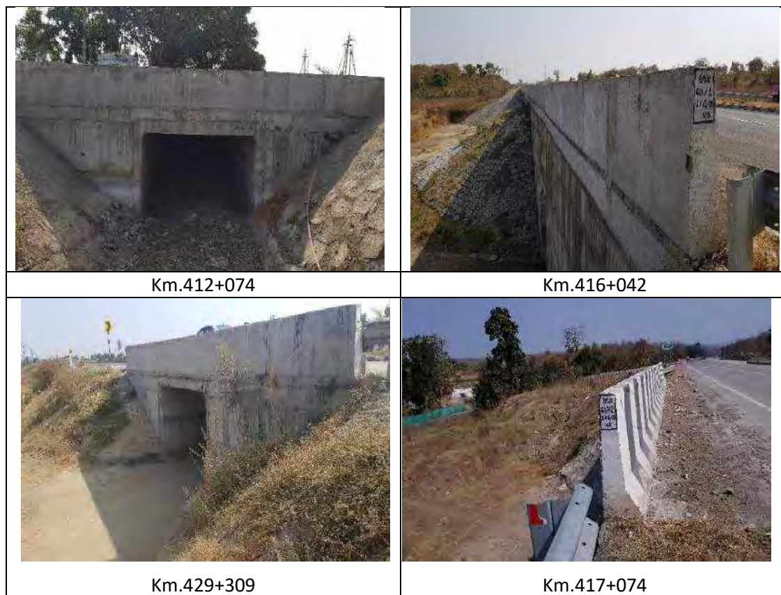
Figure 4-3: Representative photos of Slab Culverts
