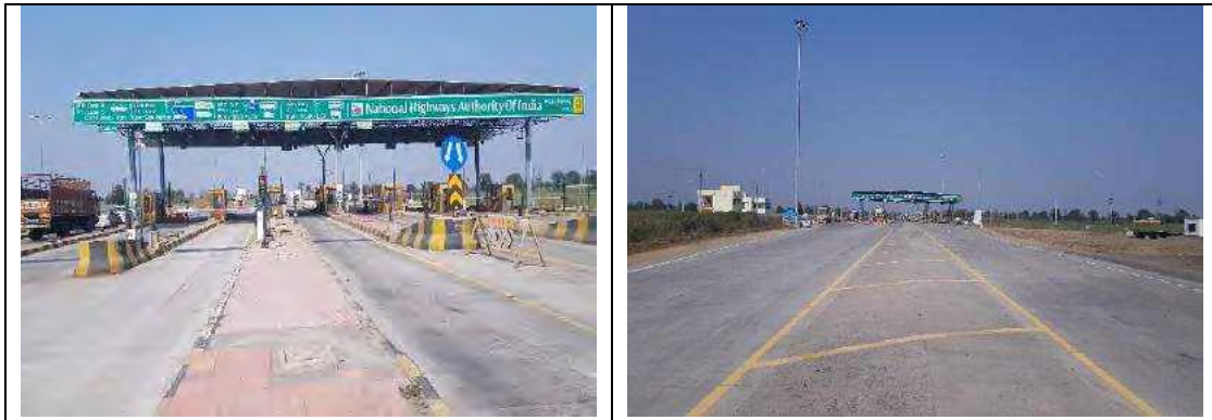
Figure 2-16: Toll Plaza at Km. 443+000
