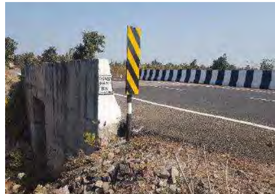
Road safety at Box Culvert at Km. 24+637
