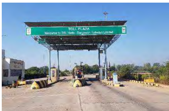
Toll Plaza at Km. 6+100
