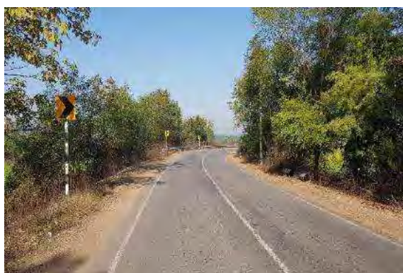
W Beam crash barrier at approaches at Km. 4+000
