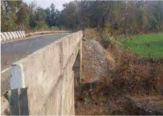
MNB approaches at Km.4+300
