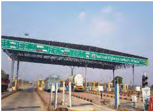
Toll Plaza at Km.382+920
