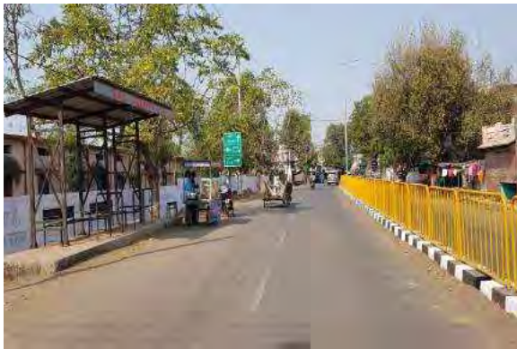
Km. 0+150 – Median Rail
