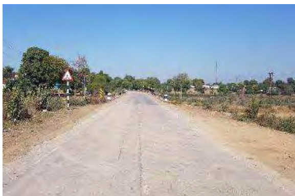
Pedestrian Crossing board at Km. 8+000
