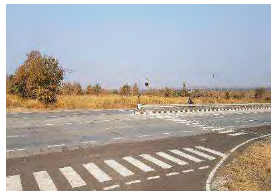
Junction at Km.392+800
