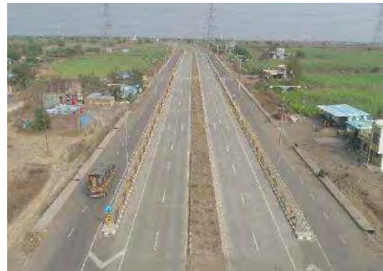
Separator Railing on Both sides at Km. 11+600
