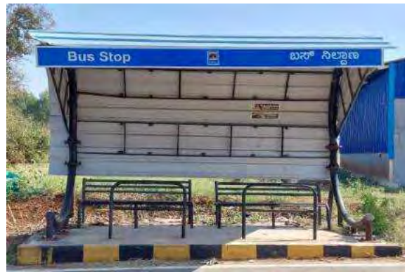
Km. 7+800 Link-B Bus Bays
