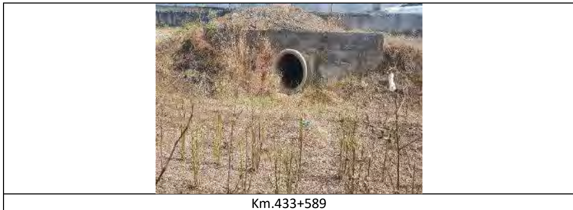
Figure 4-4: Representative photos of Pipe Culverts
