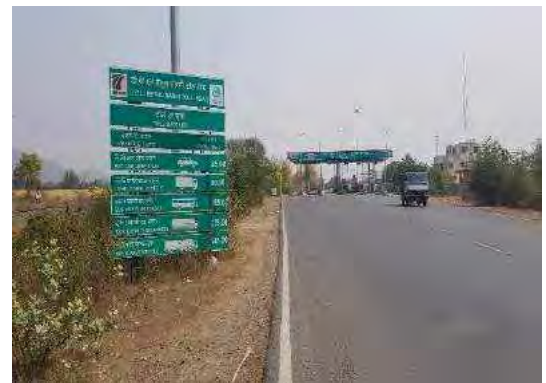
Toll Plaza board at Km. 31+000
