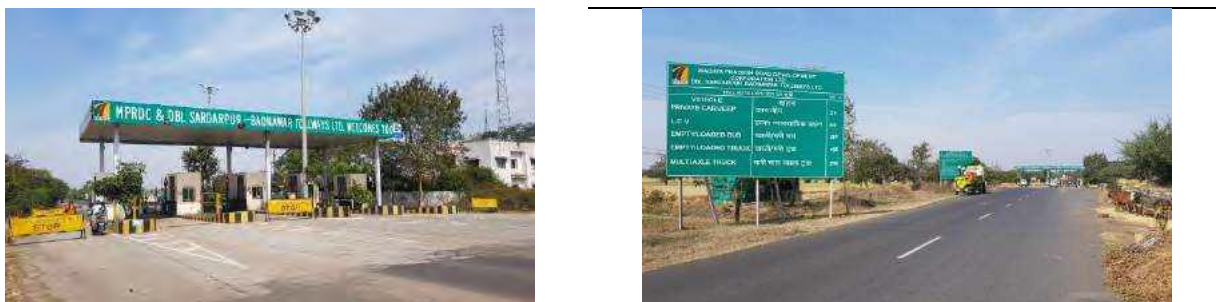
Figure 2.4: Toll Plaza at Km. 8+600
