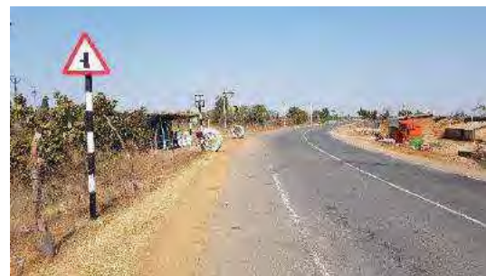
Cross Road at Km. 48+500
