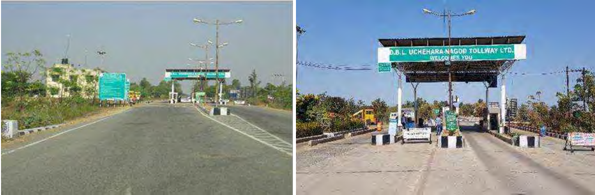
Figure 2.4: Toll Plaza at Km. 47+950
