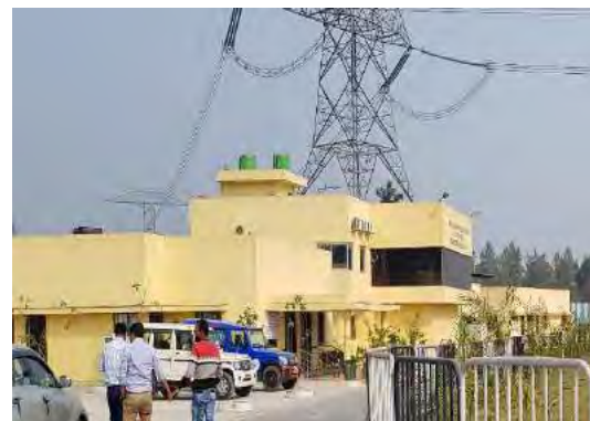
Toll Building Km. 50+900
