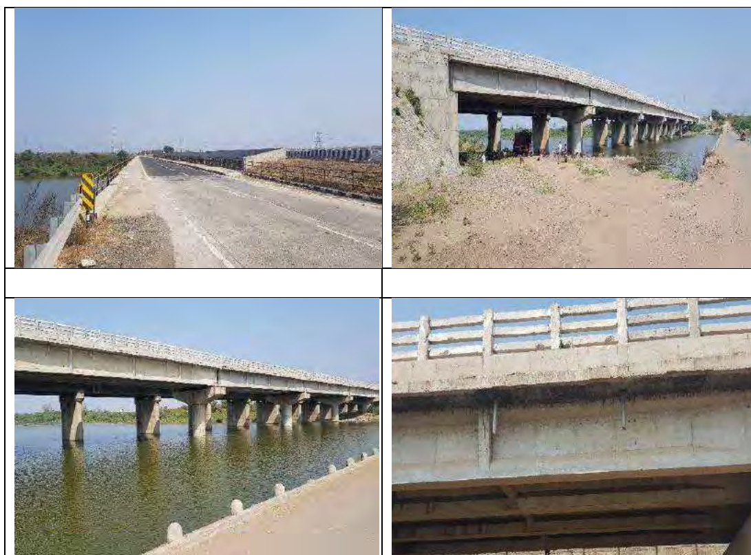
Figure 4-1: Overall view of the Major Bridge at Km. 438+813
