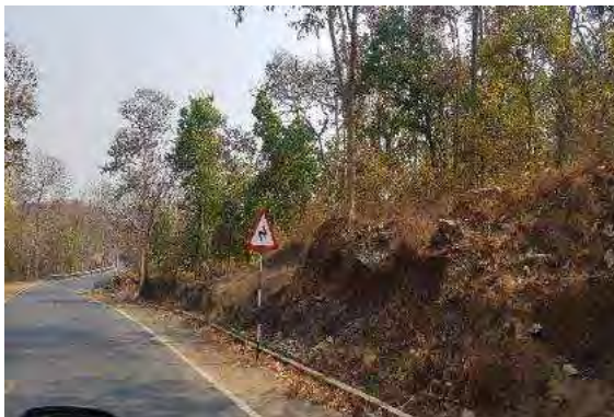
S Curve board at Km. 13+000
