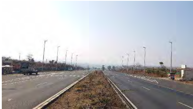
Figure 2.17: Bus bays Km. 229+700.
