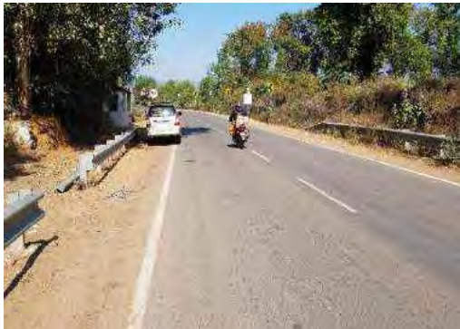
Speed Limit Board and Direction Chevron Boards
