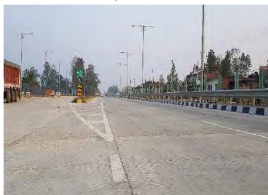
Truck Lay Bye at Km. 75+300
