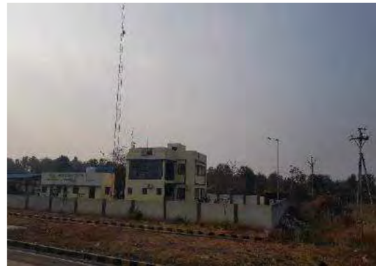
Toll Building at Km.382+920
