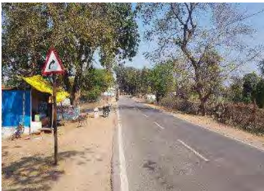
Curve Ahead sign board at Km. 48+000
