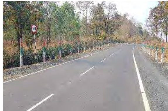
Speed Limit board at Km. 76+000
