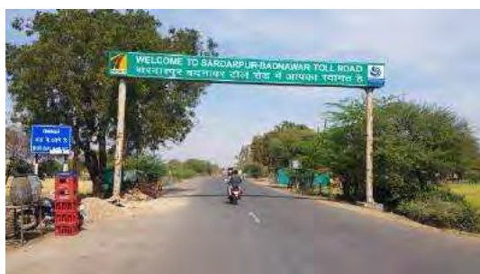
Km. 0+200 Over head sign
